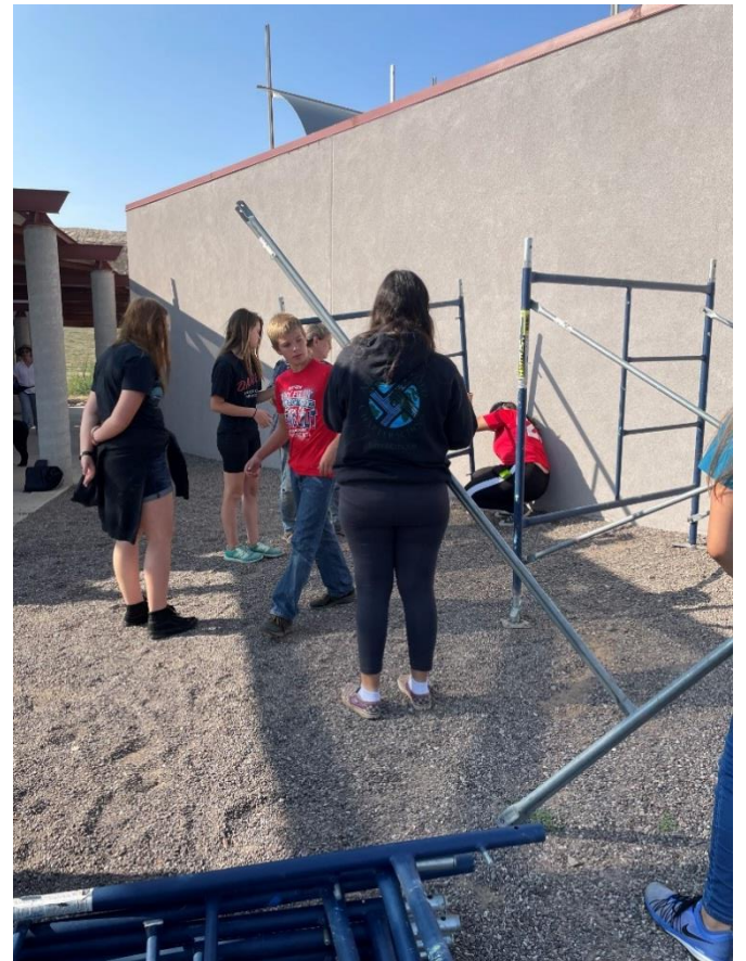
Setting up the scaffolding and preparing the wall.
